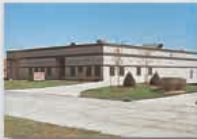
Factory Service Center - Illinois Phone 630-545-1310
